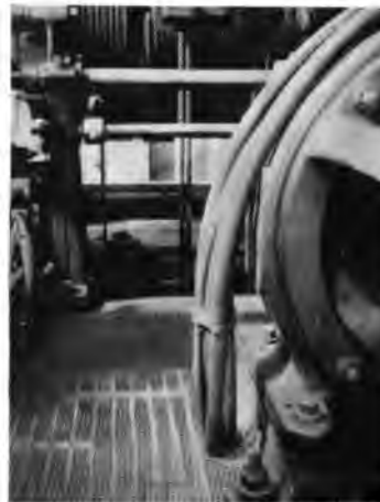
Fig. 2. Platform at Top of Shaftway.
